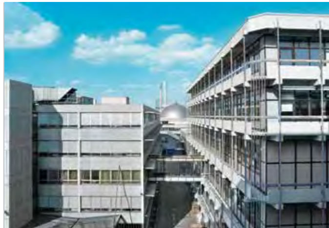
Head office Pforzheim: Reduction of pressure in the pressure network from 8.3 to 7 bar
